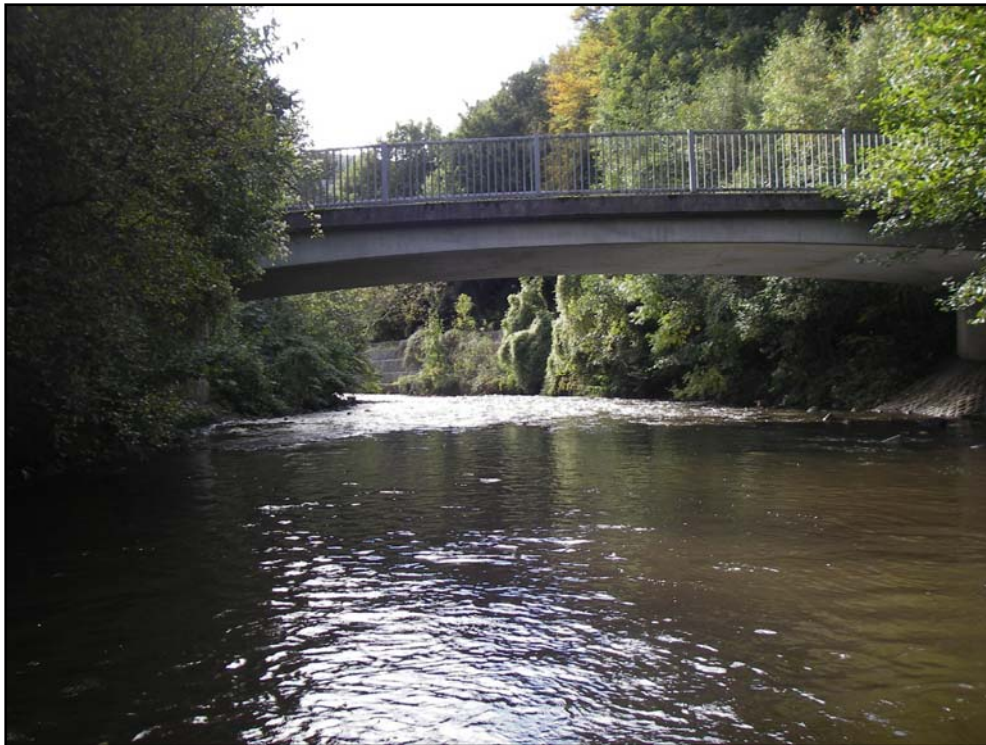
Photograph 2 – The Newport road bridge across the Afon Lwyd
