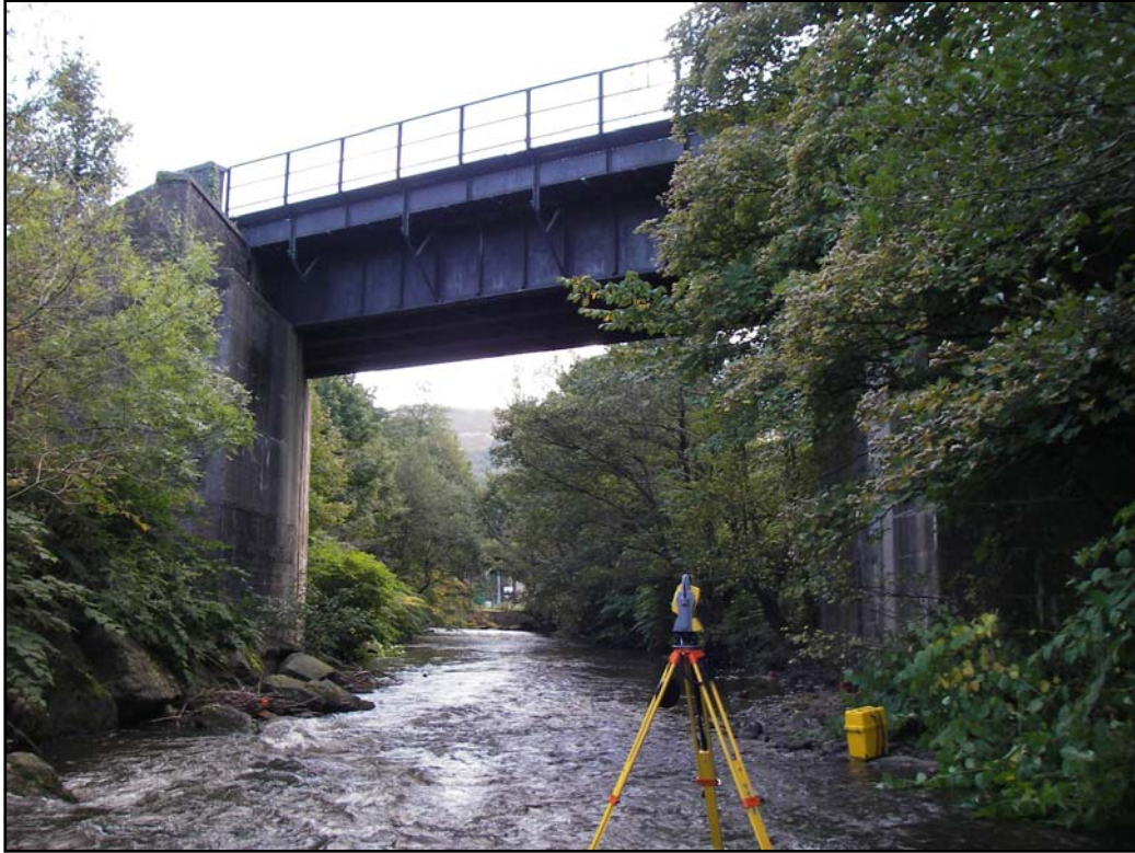
Photograph 2 – The foot bridge across the Afon Lwyd at NGR ST301989
