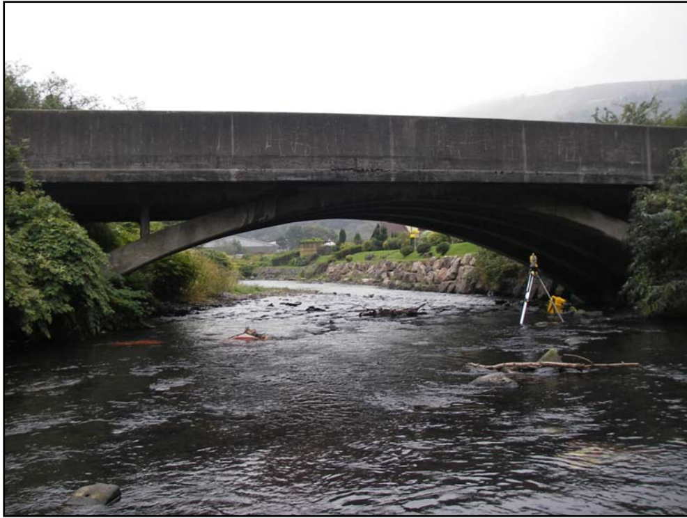
Photograph 1 – The A4042 bridge across the Afon Lwyd
