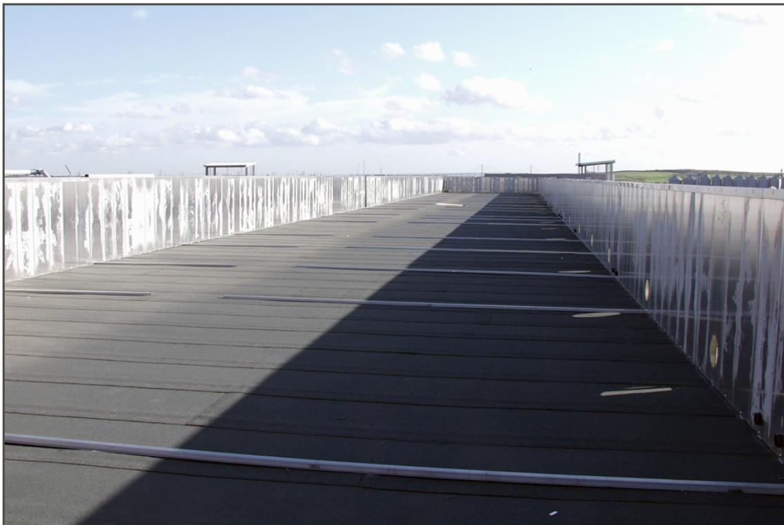
Plate 3.2: Biofilter under construction (Frog Island, October 2005).
