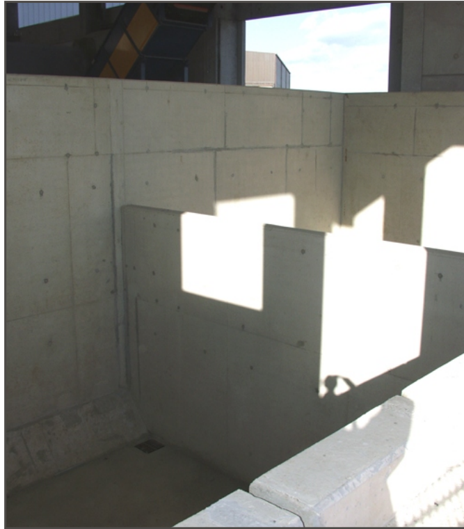
Plate 3.1: Residual MSW Reception Pits under construction (Frog Island, October 2005).
