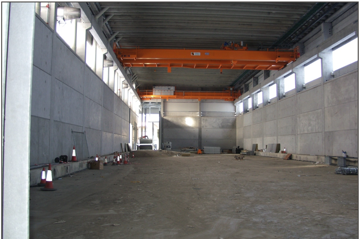
Plate 3.4: Overhead Cranes under construction (Frog Island, October 2005) within biodrying area.
